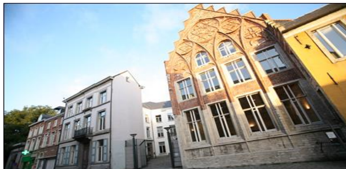
Faculty of Economics and Business - Restored historical building
